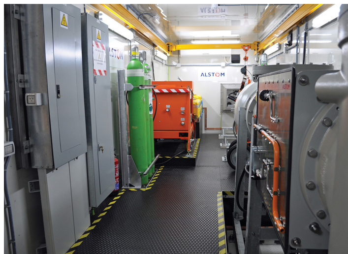
This inside view of the 115-kV mobile GIS trailer shows the AC and DC distribution panels, SF6 gas DILO cart and track-mounted crane.
