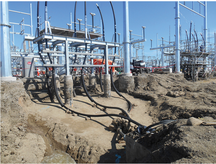
Underground cable emerging from the duct bank on the substation side during final stages of backfilling.
