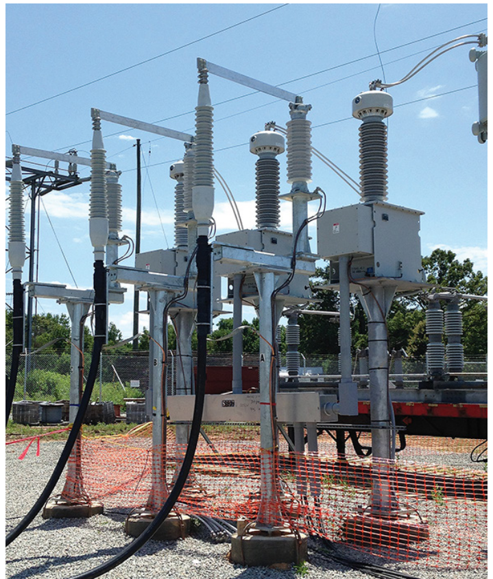
The 115-kV cable to 115-kV overhead line connection with arrestors.
