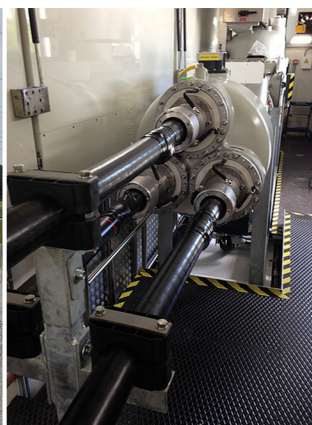
With the butterfly doors open on the 115-kV mobile GIS trailer, the GIS breaker, disconnects and ground switches can be seen. In this trailer, the 115-kV cable is not installed in this picture. However, the photo on the right shows 115-kV cables inside another 115-kV mobile GIS trailer.
