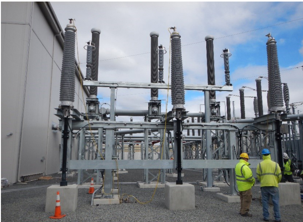
Substation terminations
