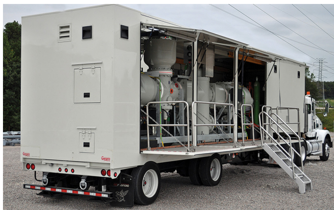
With the butterfly doors open on the 115-kV mobile GIS trailer, the GIS breaker, disconnects and ground switches can be seen. In this trailer, the 115-kV cable is not installed in this picture. However, the photo on the right shows 115-kV cables inside another 115-kV mobile GIS trailer.
