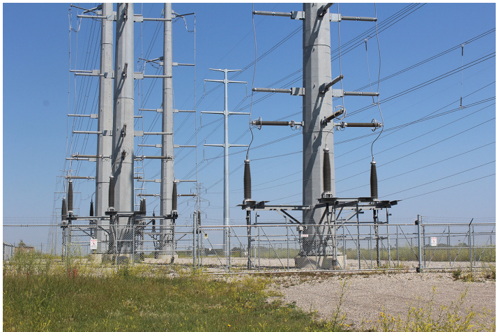
Finished riser area enclosed in a fence where 4 circuits transfer from overhead to underground to travel under the adjacent circuits to connect the new power plant to the grid.
