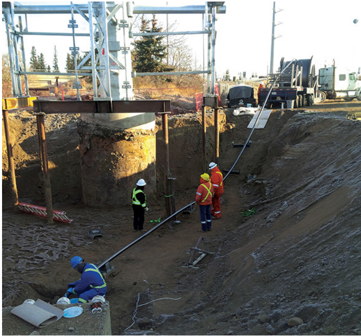
During underground cable pulling the caisson foundations are exposed which is an important factor to consider during design.
