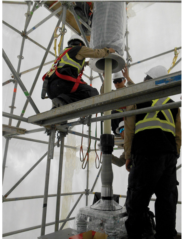
Outer bushing casing being lowered over the prepared underground cable. Once bushing has been completed it will allow the safe transition between overhead conductor and underground cable.
