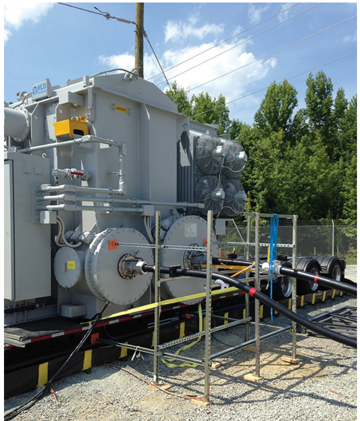
The 115-kV and 230-kV connections are going into the single-phase transformer.
