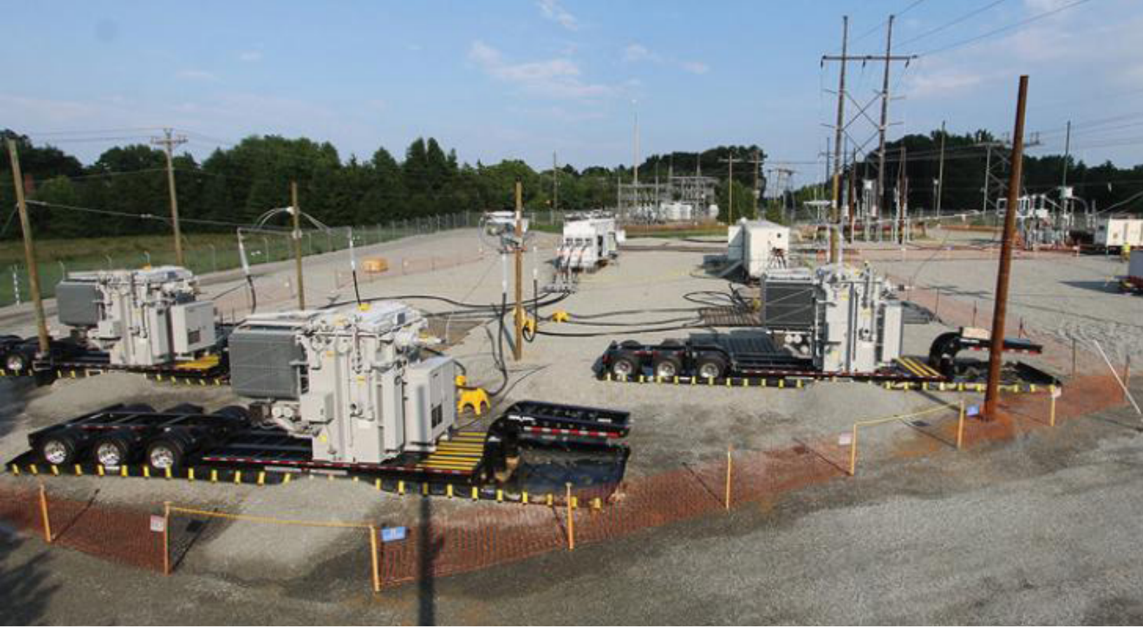
The Cartersville Mobile Substation Installation was energized in August 2016.
