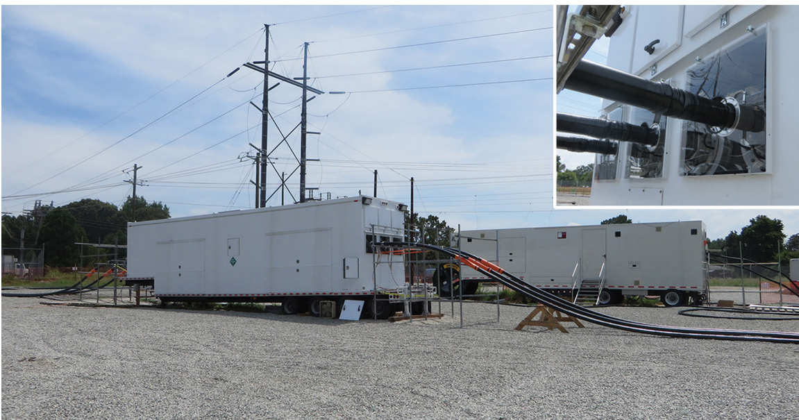
The 230-kV cables in the foreground are going into the 230-kV mobile GIS trailer, while the 115-kV cables in the background are going into the 115-kV mobile GIS trailer. The inset shows the covers Dominion Energy designed to keep animals and other elements out of the 230-kV mobile GIS trailer.
