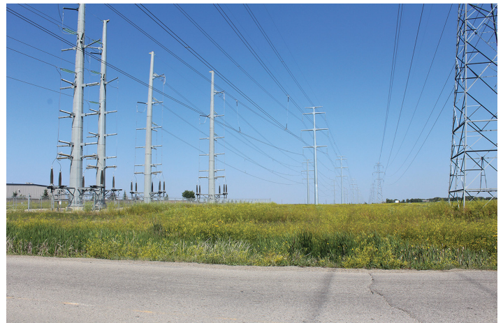
The entire transmission utility corridor (TUC) showing the new circuits transitioning to underground on the far left, a rebuilt circuit in the center, and an existing lattice circuit on the right.
