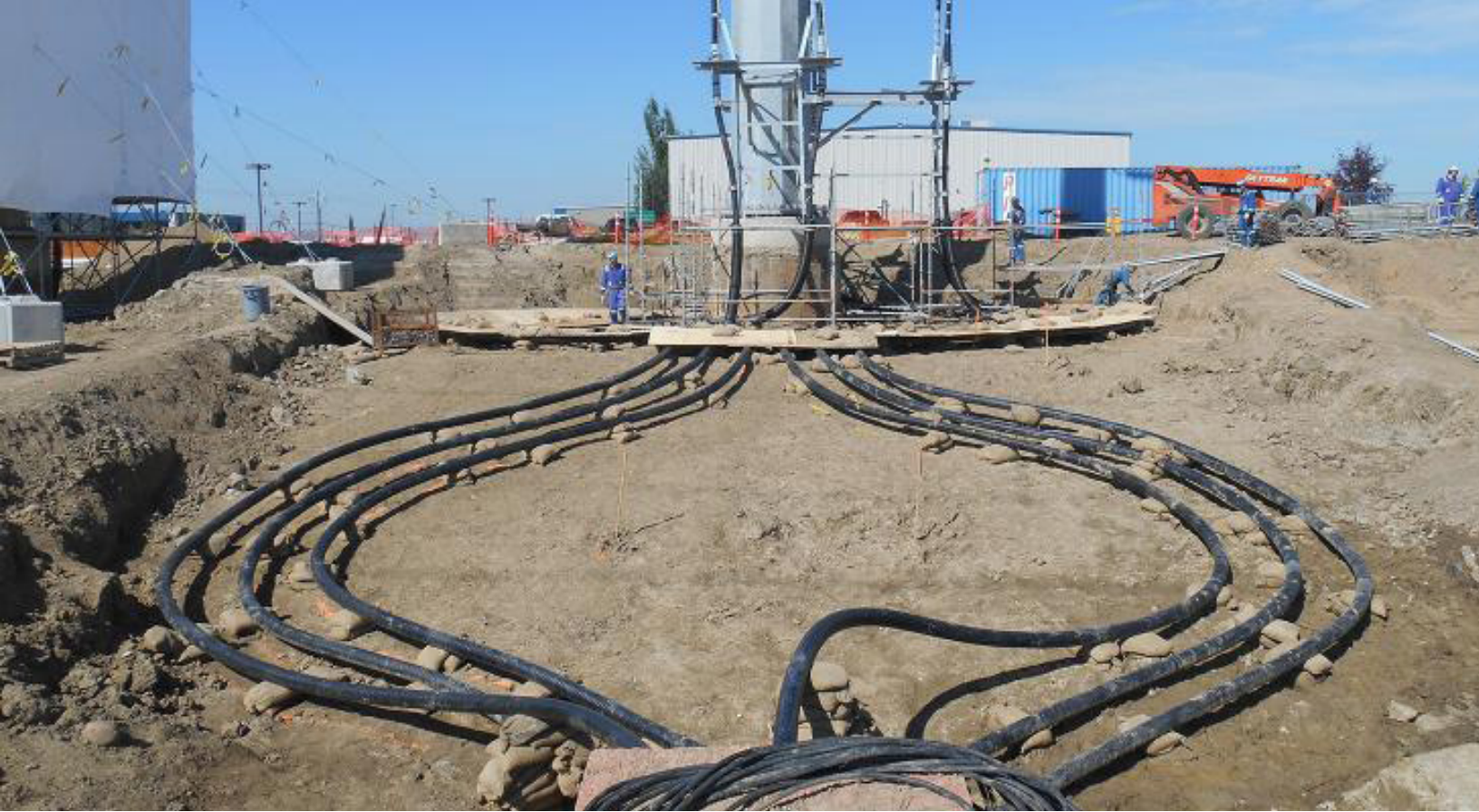
Underground cable layout showing cable loops in the direct buried section between the duct bank and riser structure.
