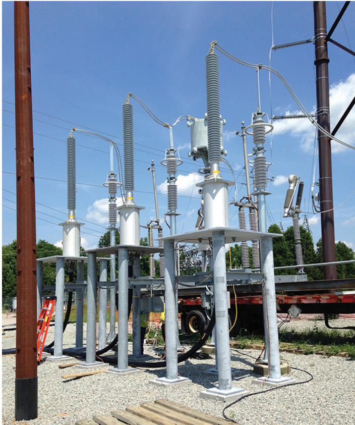
The 230-kV underground cable going into the 230-kV line connection.
