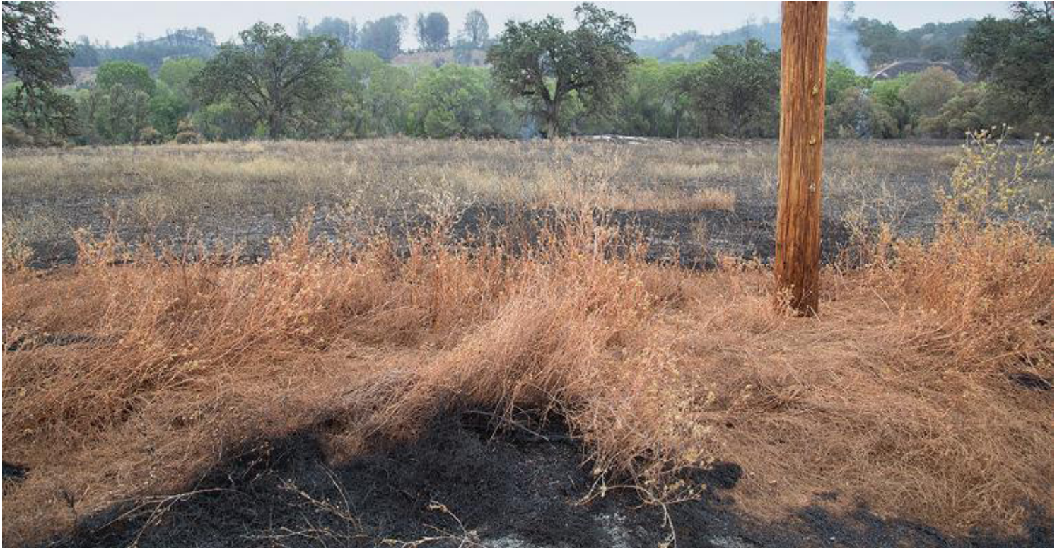
Pole and surrounding vegetation pretreated with LTR well in advance of a fire. There was no damage.
