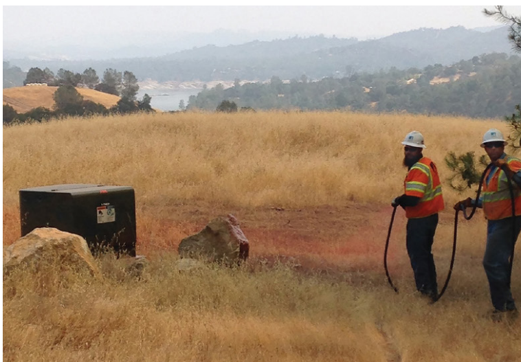
Before and after scene from 2016 fire in San Luis Obispo County. Area around pad-mounted transformer is pretreated with long-term retardant a day prior to fire burning through the area. After scene shows the effectiveness of the treatment - no damage.
