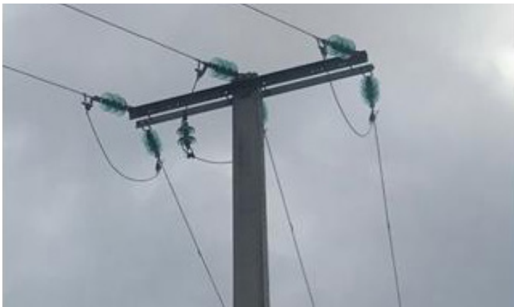
Figure 22: examples of resilient distribution lines using concrete poles and toughened glass insulators in suspension and tension.
