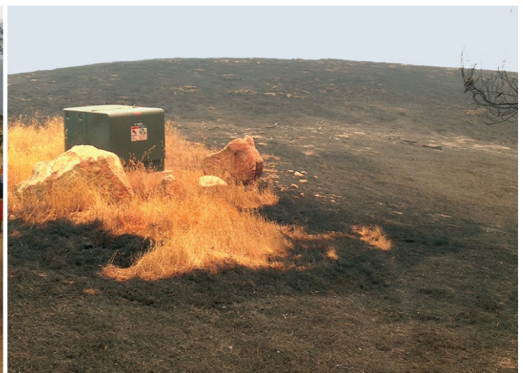
Before and after scene from 2016 fire in San Luis Obispo County. Area around pad-mounted transformer is pretreated with long-term retardant a day prior to fire burning through the area. After scene shows the effectiveness of the treatment - no damage.
