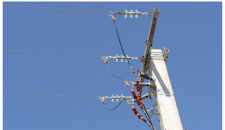
Figure 22: examples of resilient distribution lines using concrete poles and toughened glass insulators in suspension and tension.
