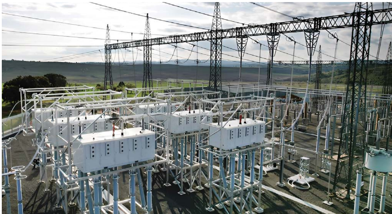
Yass substation, Transgrid continues to look at the use of modular power flow control solutions as part of its network development process. Photo courtesy of Smart Wires.
