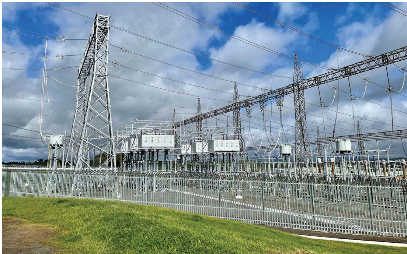
The modular power flow controllers enable real-time control of electricity flows along power lines. If the SmartValve system detects areas of congestion on the network, it can automatically redirect flows to less congested lines with spare capacity. Photo courtesy of Smart Wires.
