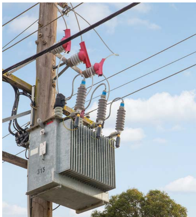
This pole-mounted SPU monitors the current and thermal load of a surge arrester and automatically disconnects it from the network in case of a thermal overload, thus preventing any arcing, sparking or ejection of hot particles that potentially could ignite a fire. Photo courtesy of Hitachi Energy.
