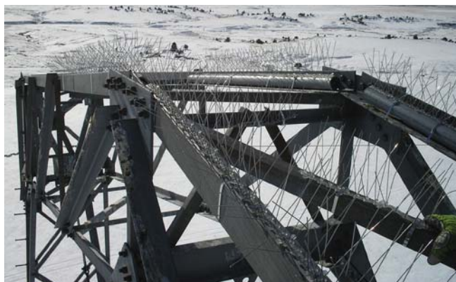
Perch deterrents installed on a 500kV tower. Photo by NorthWestern Energy.
