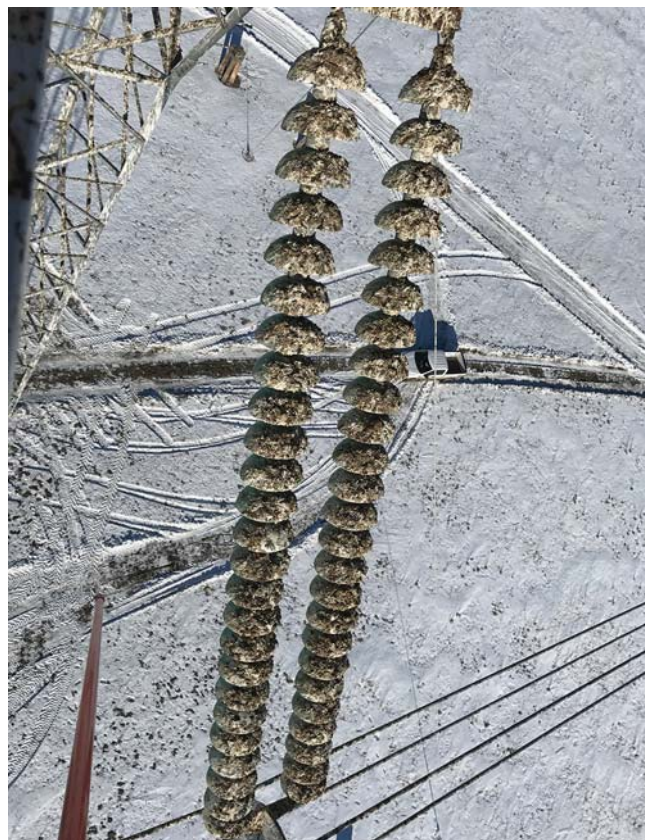
500-kV insulators heavily contaminated with bird droppings and pellets. Photo by NorthWestern Energy.
