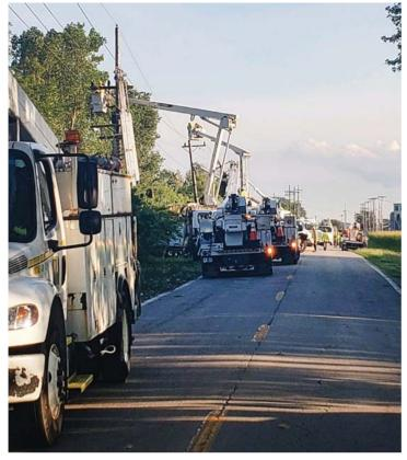
Bucket trucks lift workers and equipment to repair and replace utility poles and cross arms shattered by a storm. Photo by ComEd.
