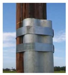
Steel trussing is commonly used for network hardening as well as pole restoration. Photo by NESC.
