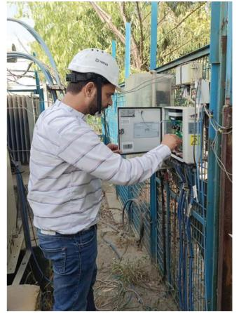
Low-voltage IoT device installed in outdoor substation. Photo by Tata Power.
