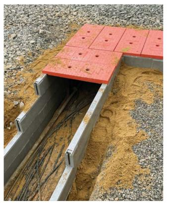
To repair these types of trenches, contractors typically remove the trench and in the process disturb the cables. Individual pieces of STAKKAbox were repurposed to make a trench that was high strength while also being lightweight and flexible.
