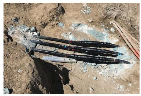
Onsite repair of splices that had been exhibiting PD and were performing below manufacturer's standards. IMCORP's PD test confirmed repaired splices were PD free to 2.0Uo. Photo by IMCORP.
