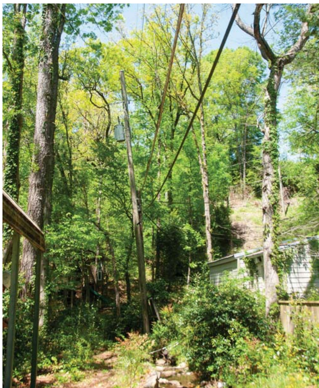
The Green Valley undergrounding project was a challenge from both a size and complexity perspective. Nearly 8,000 feet of overhead was located rear of customer properties serving 101 separate meters. Photo by Alabama Power.
