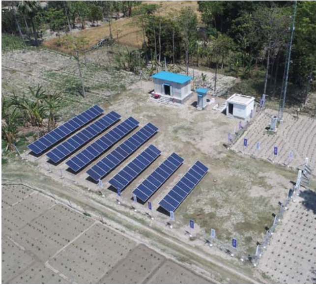
Aerial shot of a mini-grid under construction in Aurai, India. Husk's mini-grids are located close to main market areas, and distribution networks need to cover 80% of commercial customers to maximize both local impact and company revenue. Photo by Husk Power.
