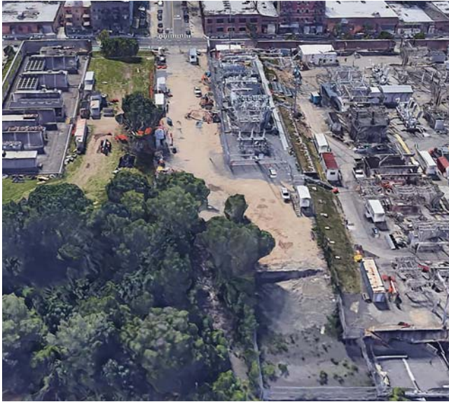
An aerial shot of Con Edison's Rainey Substation in Queens. The utility budgeted US$275 million for T&D projects in Queens, but now expects to save $40 million. Photo courtesy of Con Edison.
