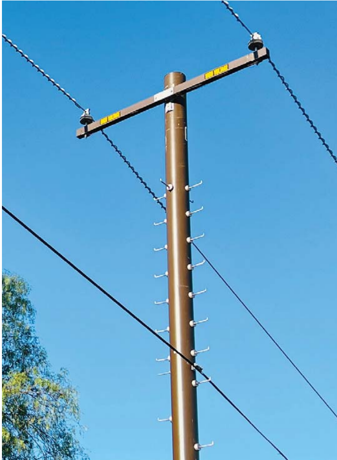
FRP poles have been used for 25 years in the industry, with success and reliability. FRP is as suitable for utility poles as steel, concrete and wood.
