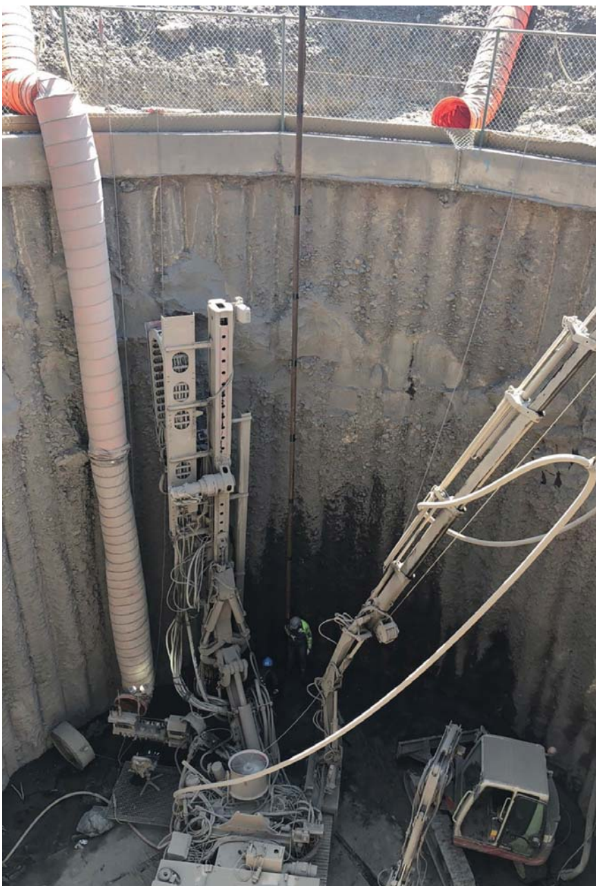
Construction of one of the access shafts of the tunnel under the Meuse River and Albert canal: installation of concrete pilings to stabilize the surrounding soil and allow digging to occur. Photo courtesy of Elia.
