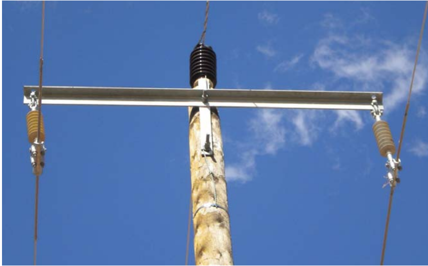
Example of a typical steel cross-arm. Photo by Eskom.
