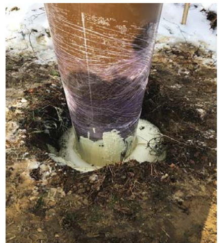
Backfilling of poles with foam. Courtesy of SMECO
