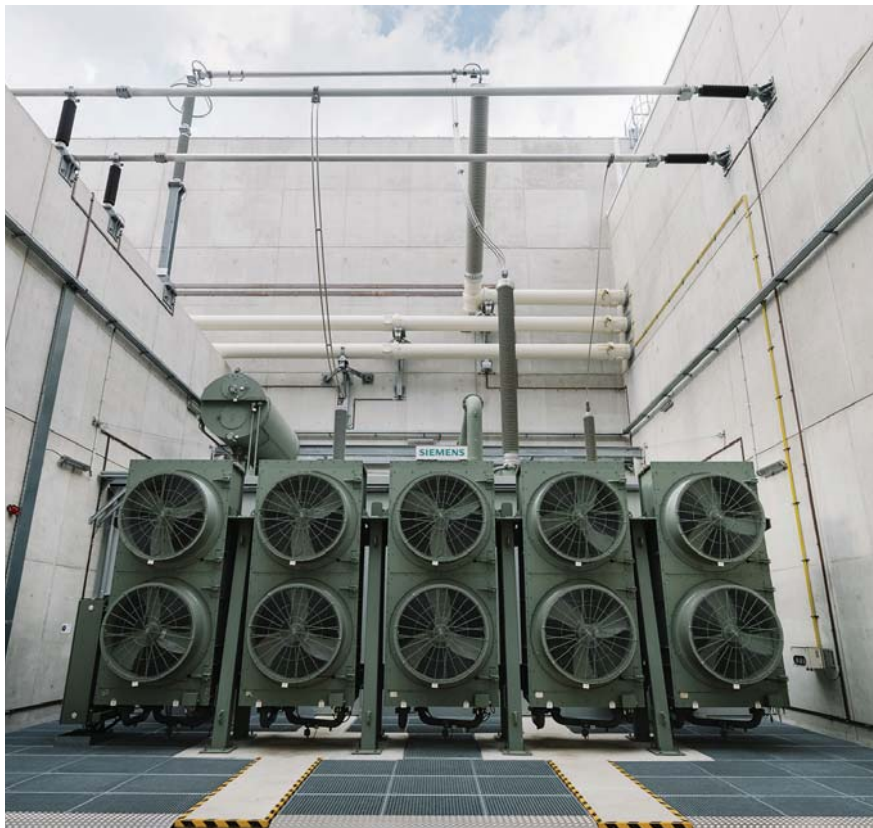
One phase of the converter transformer, which ensures that the converter gets the required voltage, irrespective of the voltage fluctuations of AC networks. Photo courtesy of Elia.
