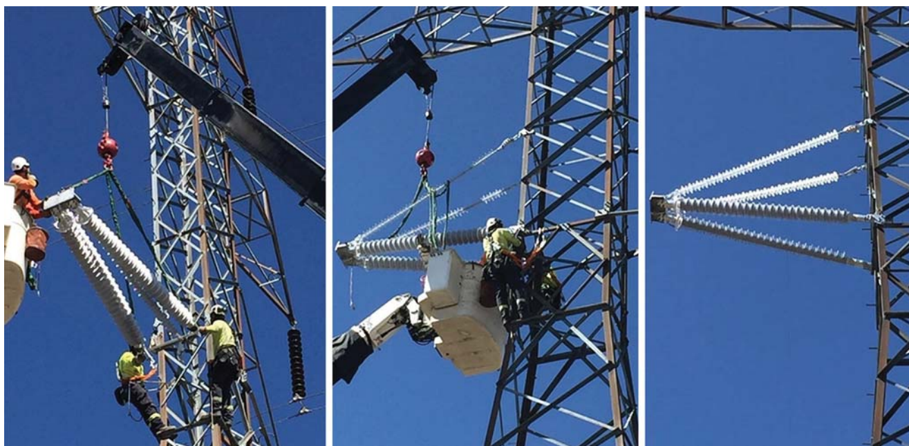
Composite insulated cross arm (CICA) field installation. Courtesy of AltaLink.
