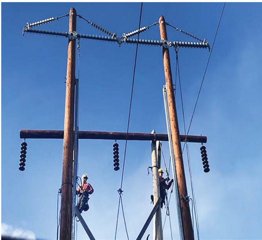
Totally insulated framing (TIF). Courtesy of AltaLink.
