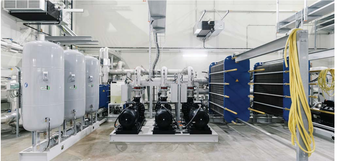
Pumps belonging to the water cooling system that release the switching losses of the converter using a combination of demineralised water and glycol water. Photo courtesy of Elia.
