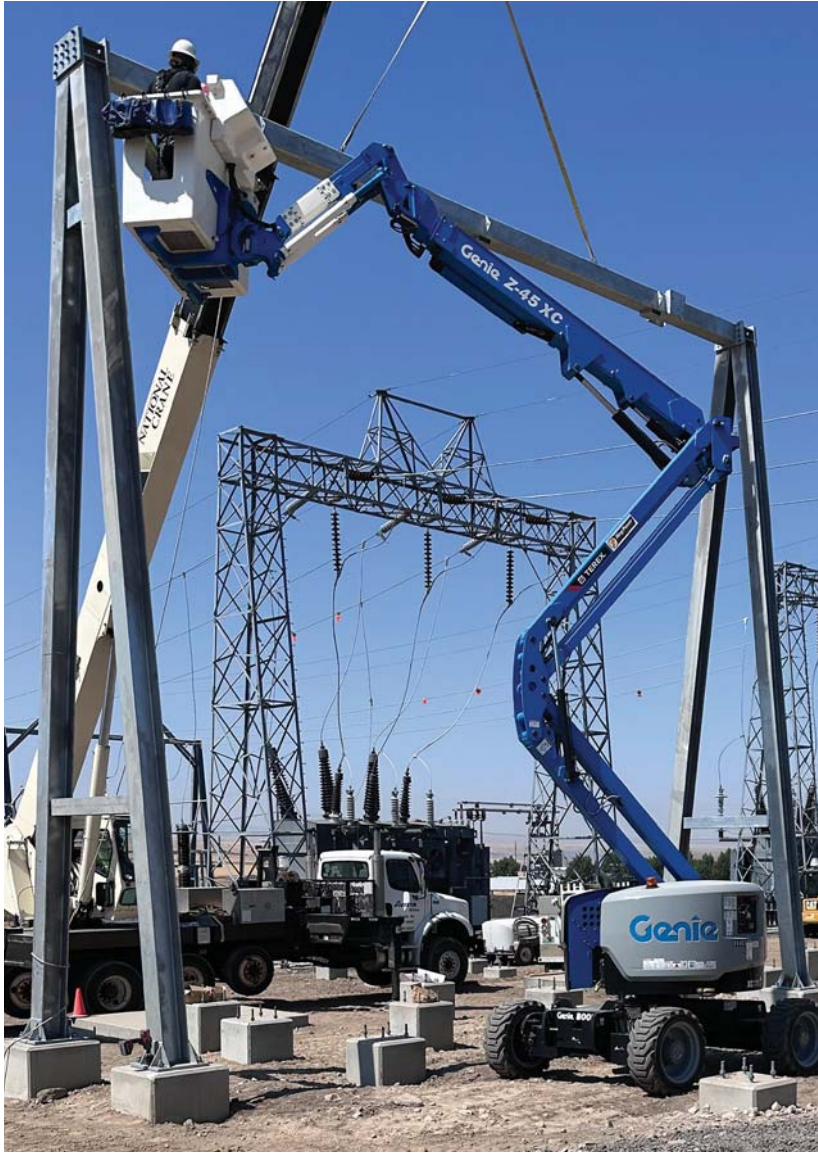
Avista workers found the safety features of this equipment enabled them to work with insulated equipment without sacrificing speed and side cutouts in the insulated bucket provide line of sight visibility to workers on the ground. Photo by Avista Utilities.
