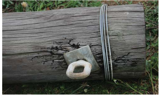
Example of a bonded cross arm. Photo by Eskom.
