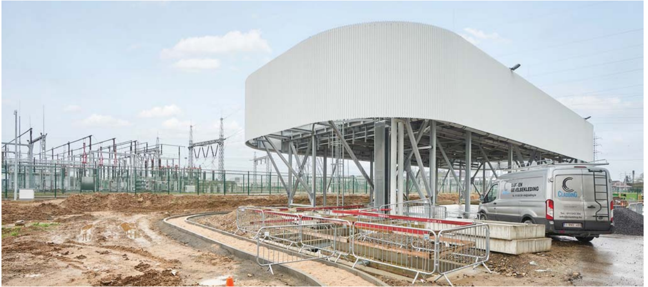
Dry outdoor cooler where the switching losses of the converter are released. Some of the losses are captured and used to heat the building.
