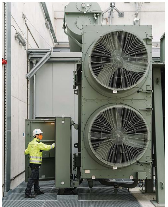
Technician inspecting the cooler bank of one of the converter transformers. Photo courtesy of Elia.
