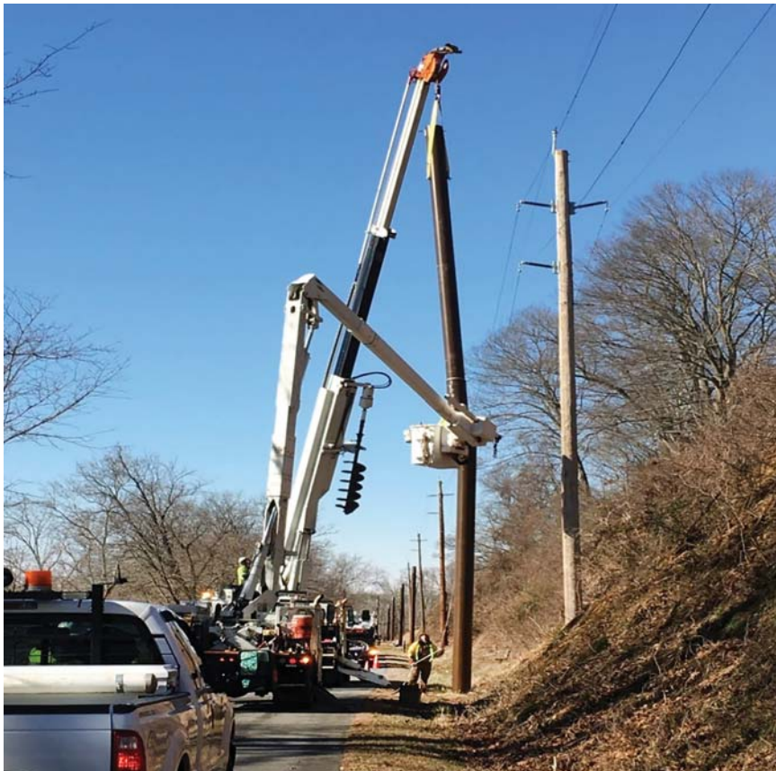
Lifting the pole top into place with line energized. Courtesy of SMECO.
