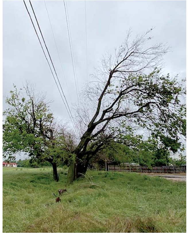
Low-volume spray trim applications in the wire zone allow OG&E to control only portions of trees that pose a threat to impact overhead power lines. Photo courtesy of OG&E.
