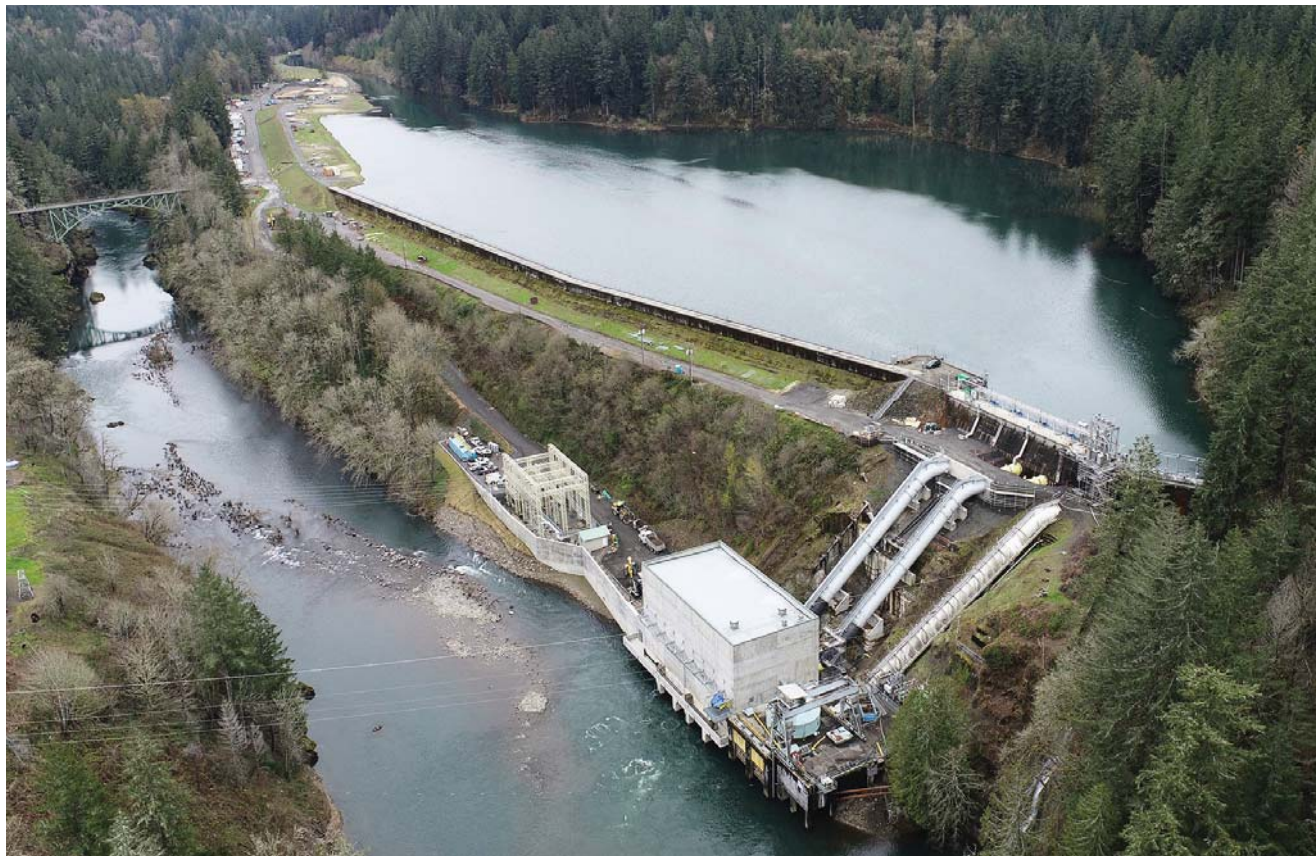
In addition to procuring wind, solar, and battery storage, PGE is also investing in the performance of its hydropower projects, including the recently modernized Faraday Powerhouse – a 116-year-old hydropower facility on the Clackamas River. This multiyear restoration effort improved the efficiency and seismic safety of the historic plant. Photo courtesy of Portland General Electric.
