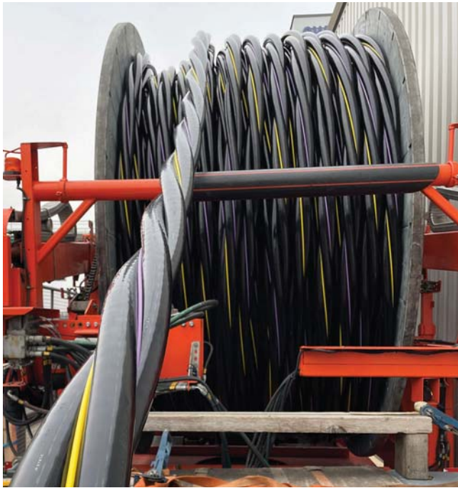
150-kV three-core cables before installation. Photo courtesy of ewz.
