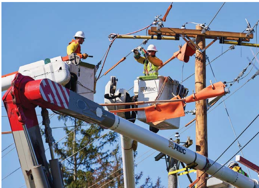
In Ohio, FirstEnergy contractors perform work at height on the utility's Grid Mod I set of system upgrades. Photo by FirstEnergy.
