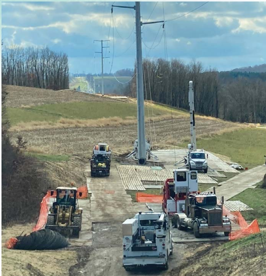
American Transmission Systems, Inc. (ATSI), a subsidiary of FirstEnergy Corp., works on upgrades to 13 miles of a high-voltage transmission line in Carroll and Columbiana counties in Ohio. Upgrading this segment was the first phase of a larger 64-mile transmission line project. Photo by FirstEnergy.
