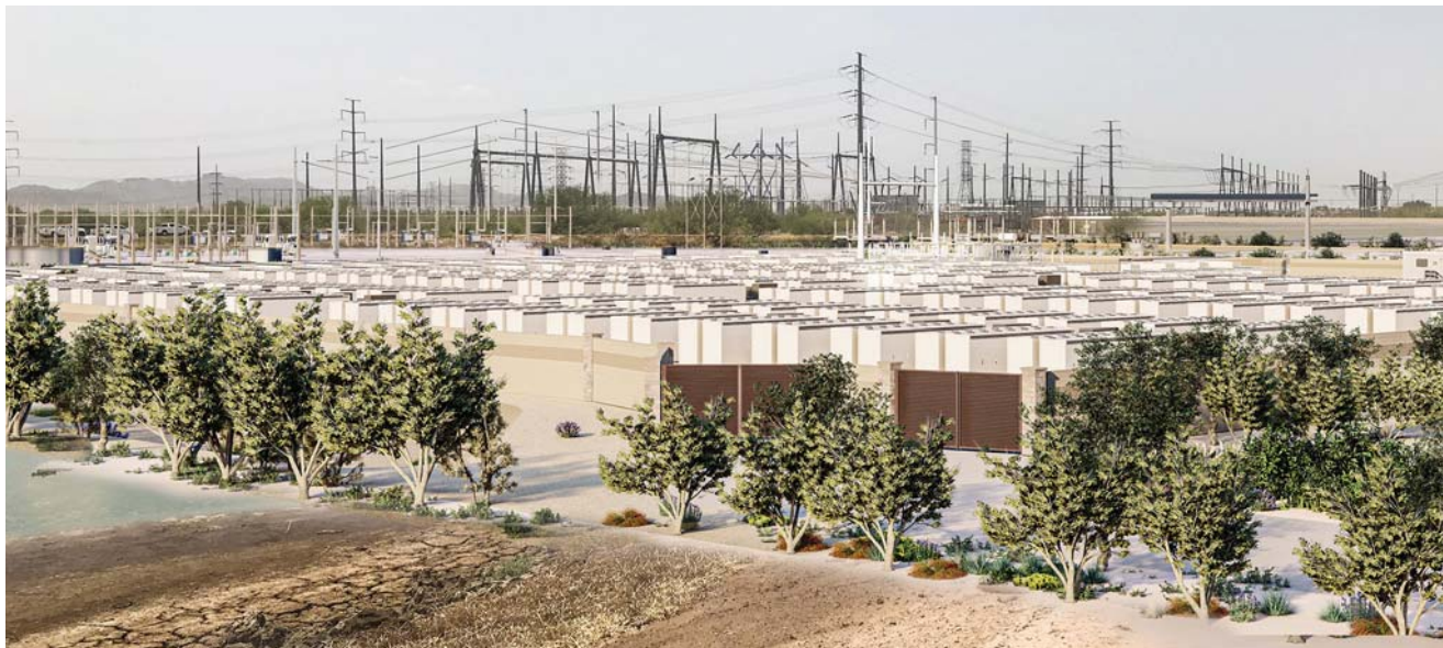
Plus Power rendering of the Sierra Estrella battery storage system to be located in Avondale, AZ. Photo by Plus Power.
