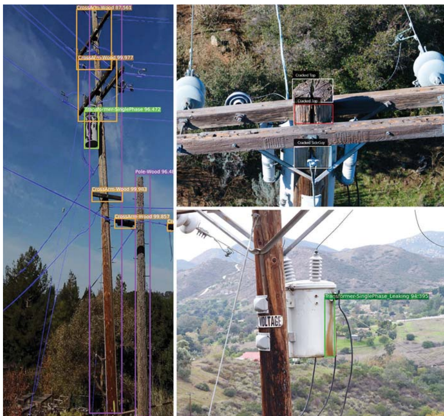
A feedback loop was created within the platform, enabling qualified workers to validate machine learning results to optimize the model performance. The team built a map-based user interface to visualize and browse for imagery and machine learning results stored in the image repository. This helped the utility to identify additional issues to repair, leading to a more effective inspection program. Photos by SDG&E.
