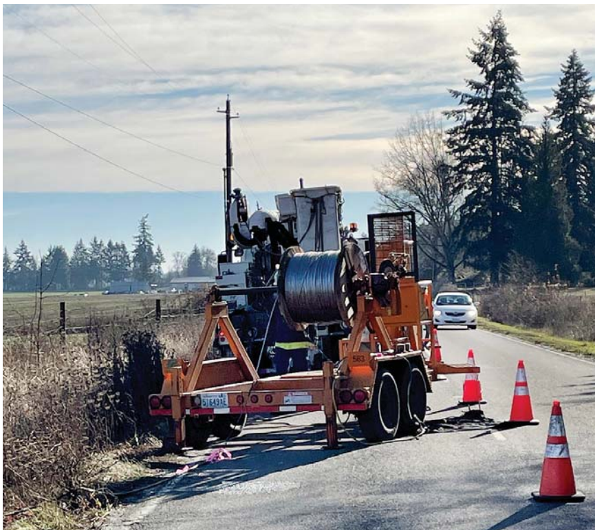
New conductor ready to install in the Willamette Valley. Photo by Portland General Electric.
