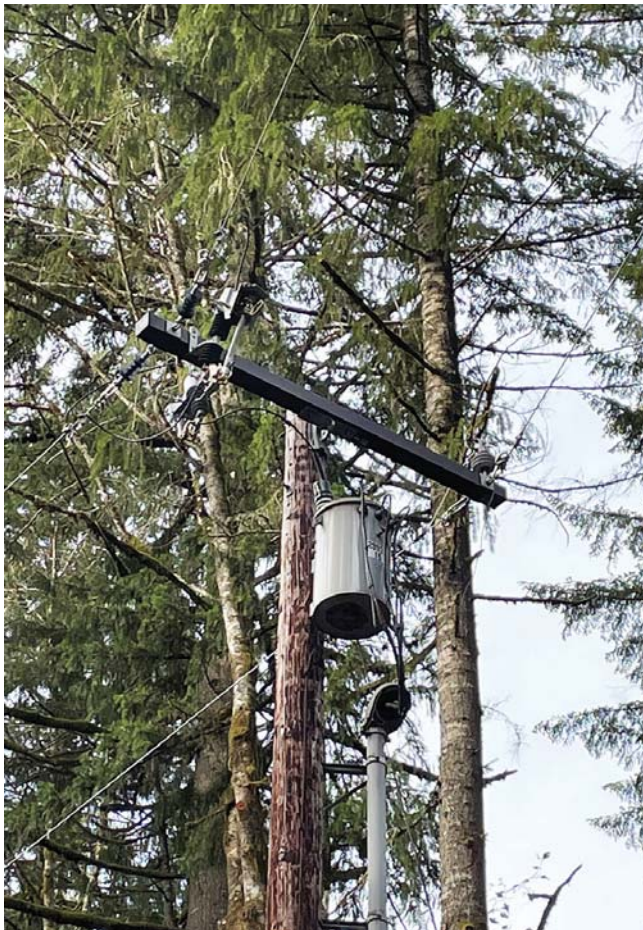
A power pole equipped with a new conductor, X-arm and cutouts. Photo by Portland General Electric.
