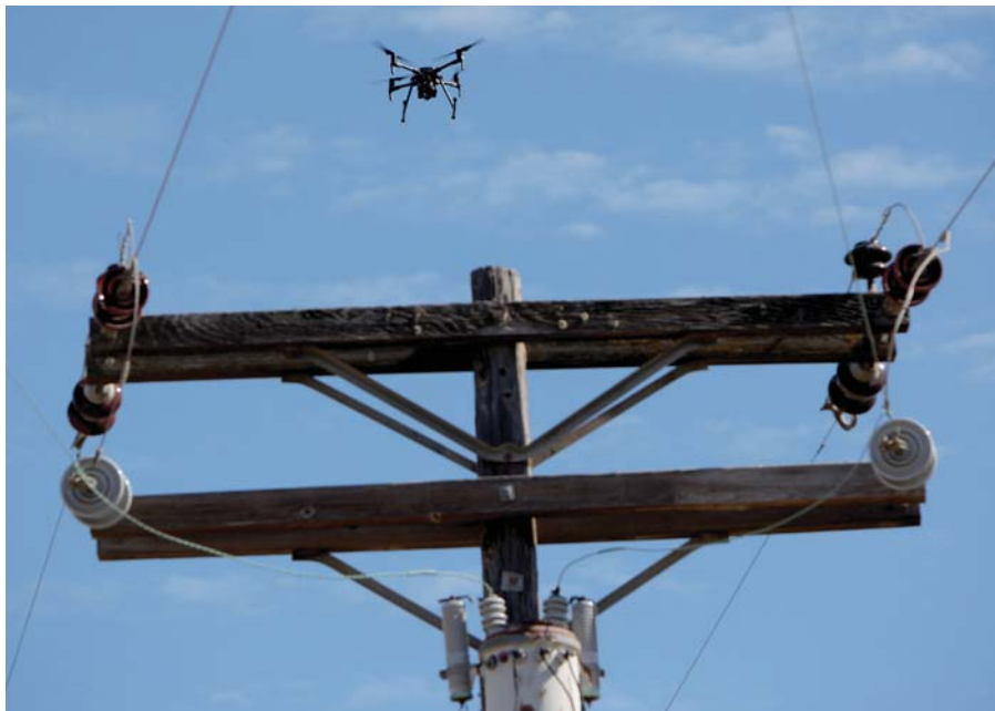
The advantages of drone inspections over ground inspections were quickly realized, including the top-down and close-up views drones provided. Photo by SDG&E.
