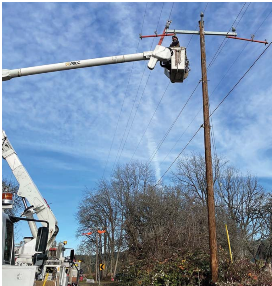
A utility worker clips in a new conductor to a distribution crossarm. Long-term system hardening projects — including overhead-to-underground conversion, covered wire and intelligent reclosers — are critical to the reduction of wildfire risk. Photo by Portland General Electric.
