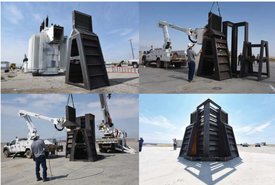
The Idaho National Laboratory developed the Armored Transformer Barrier after the 2013 Metcalf substation attack, and it has since been licensed for production. The barrier is made of military grade steel that is "inexpensive, yet rugged," according to the laboratory. It was tested to defend critical infrastructure from explosives as well as high-powered firearms, as well as natural disasters like a Category 2 hurricane. The design is modular and can be shipped disassembled before being installed with common hand tools, utility cranes and forklifts. Photo by Idaho National Laboratory.
