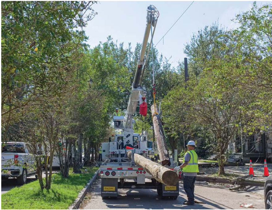
Heavy equipment delivers new distribution poles to workers performing outage restoration. Having a centralized tool with standardized processes for each project team to contribute to and work from helps create a clear picture of project progress and allows issues to be elevated efficiently and in a timely manner. Photo by William Morgan, Dreamstime.
