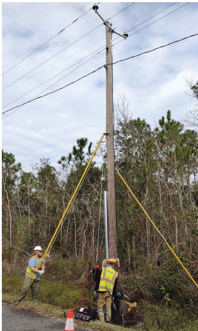
Osmose crews installing a Tough Truss Extra to restore and strengthen a pole as part of a resiliency program Photo by Osmose.
