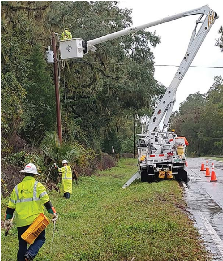
Line crews from Duke Energy's Wildwood Operations Center in north-central Florida work to restore power to a neighborhood in Sumter County, Florida.
