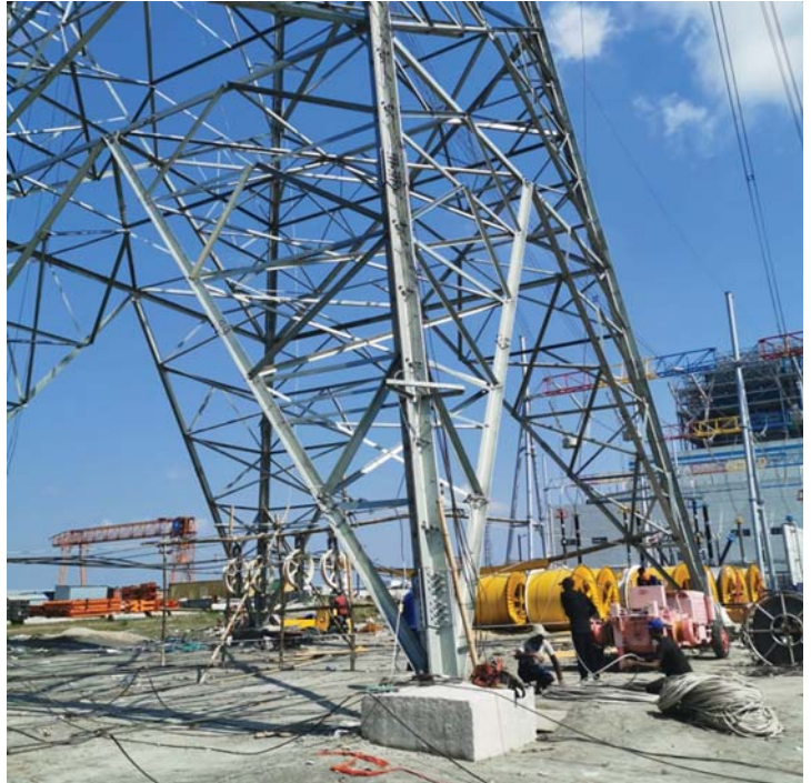
Conductor stringing works near Gopalganj substation.
