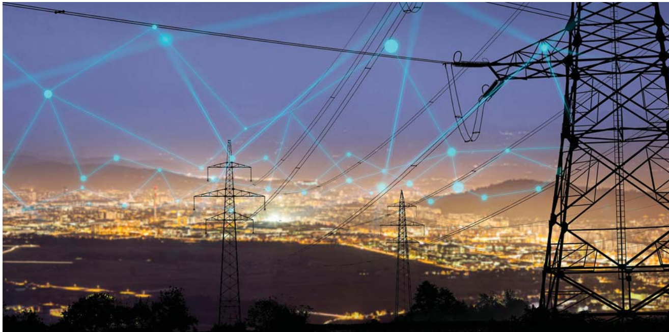
Photo courtesy of Hitachi Energy
