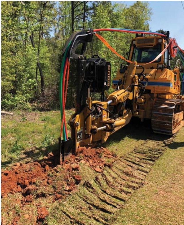
Long-haul communication thoroughfares connect major hubs, cities, towns, generation plants and substations. These new underground routes are in addition to existing and new OPGW projects on the transmission system, and they will eventually cover much of the state. Photo by Alabama Power.
