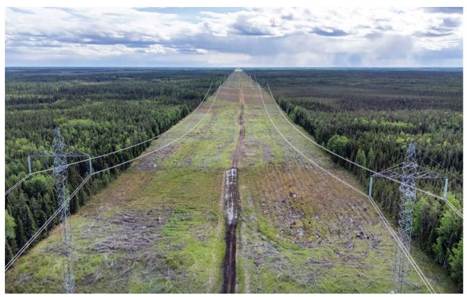
By measuring the distance to the vegetation from the fitted curve, Manitoba Hydro discovered the closest point between the vegetation and the curve was about 15 ft to 18 ft at the time of the event, which exceeds industry requirements.
