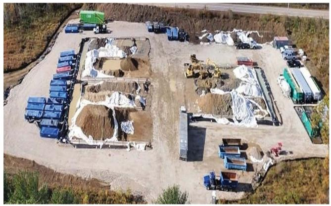
Crews collected more than 22,000 tons of soil and disposed of contaminated dirt. No contaminated soil was returned to the ground. They also collected and treated around 385,000 gal (1750 cu m) of water. Photo courtesy of Eversource
