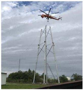
A heavy-lift helicopter, the Erickson Air Crane, was used to set the poles for the transmission structures which were built in sections. Photo by  $\mathsf{Cleco}$
