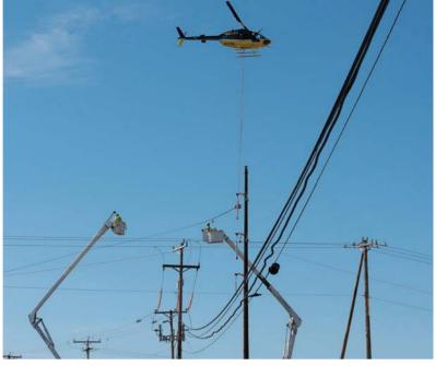
The overhead design and construction used various configurations and installation techniques including spacer cable distribution underbuild and helicopter rope installation to limit visual and construction impacts.
