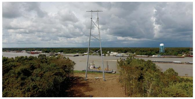
One of the new steel transmission structures built during the project. The largest structures are approximately 239-feet tall, the equivalent of a 22-story building. Photo by Cleco.
