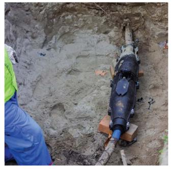
A worker repairs a cable sheath on a power cable installed in the 1970s. As discussed in the first part of this series, repairs on average underground cables can be more time consuming and expensive than those on average overhead lines. Photo by Spettacolare, Dreamstime
