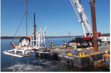
While hydroplowing is a common technology and industry practice for cable installations in water crossings and estuaries, hydroplow installation had never been used in New Hampshire.
