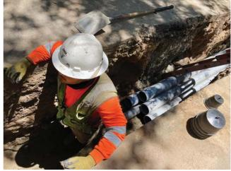
PG&E contractor runs conduit ranging in diameter from 2 inches to 6 inches, depending on cable. This project helped with system hardening and wildfire mitigation, but also improved reliability for approximately 11,000 customers.
