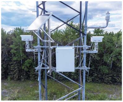
At five locations with historically active unexplained flashovers, Manitoba Hydro installed a cabinet with computer hardware and batteries, cameras, lidar, environmental sensors, solar panel and a satellite dish for system monitoring and remote data transfer.
