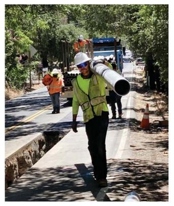
Schedule 40 PVC conduit encased four 12-kV circuits in open trench. Now that the lines serving those customers are underground, the risk of a fire from vegetation contact with overhead conductors has been mitigated and the customers have not been impacted recently by PSPS events.
