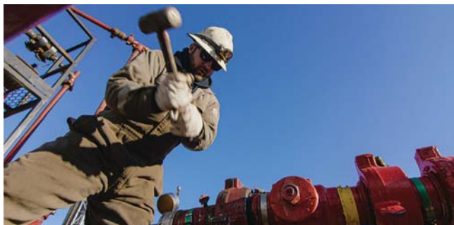
During the storm, natural gas production was interrupted by wellheads becoming frozen or having mechanical failures caused by cold weather. Texas generates nearly 45% of its electricity from natural gas. Photo by Getty Images
