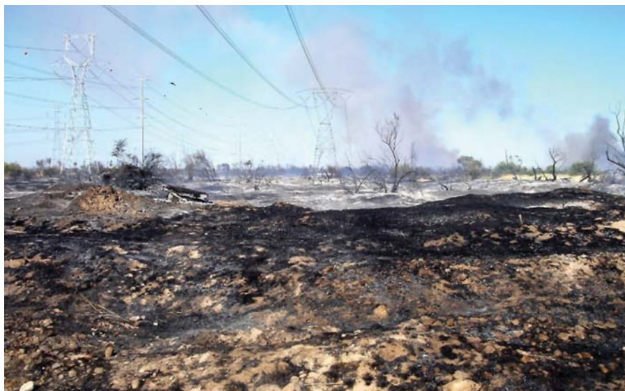
June 2005 wildfire in Phoenix, Arizona, causing outage on six circuits of 500-kV, 345-kV and 230-kV transmission lines. Photo courtesy of the authors
