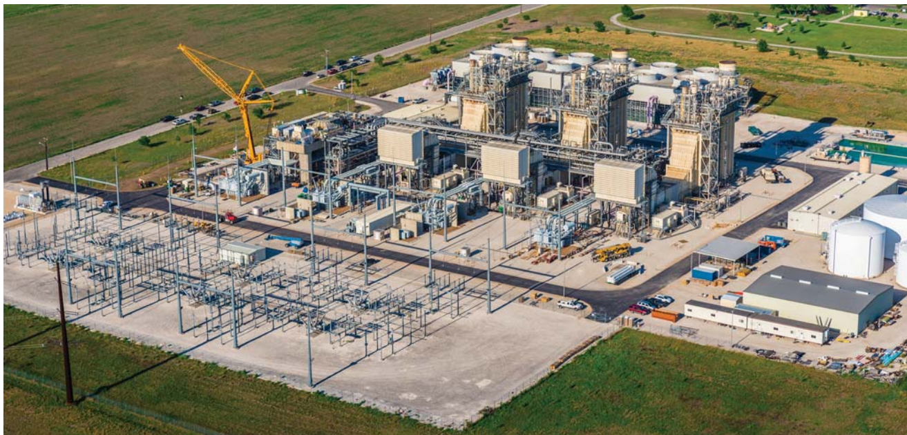
Texas natural gas combined cycle power plant. The Texas PUC has enacted penalties for power plants that do not winterize and are inspecting plants to ensure weatherization upgrades are installed. Photo by Getty Images
