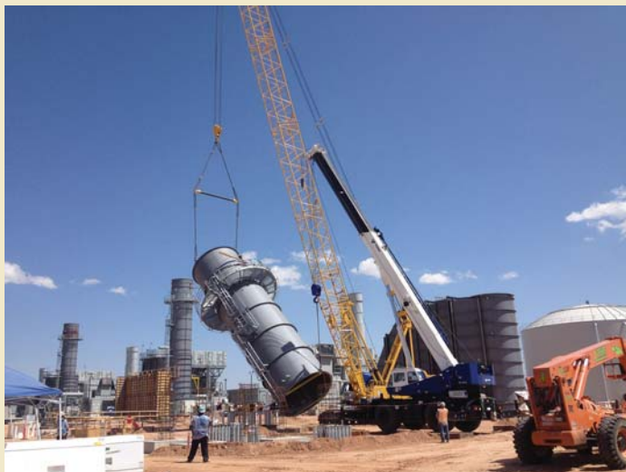
Construction at El Paso Electric's natural gas-fired Montana Power Station. The station was upgraded after a 2011 cold weather event to have quick-start capability for better power grid stability. Photo by El Paso Electric
