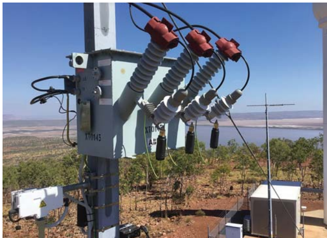
SPU devices deployed on a utility pole in the field (left); Hitachi Energy's Spark Prevention Unit (SPU), (right). Photos by Hitachi Energy.
