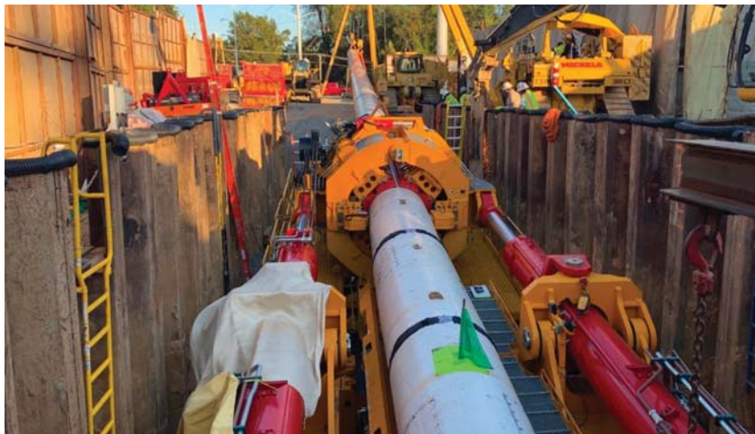
The launch pit for the Direct Pipe solution. Project partners found that Direct Pipe was the best method to reduce the risks of inadvertent return events. Photo courtesy of Dominion Energy.
