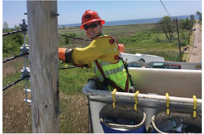
Journeyman Lineman Rick Soto says during storm restorations, it feels great to help others in need.
