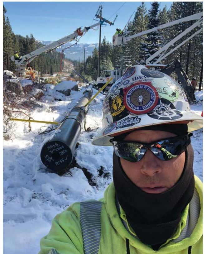
As part of his training through the International Brotherhood of Electrical Workers (IBEW), Joe Robertson has dead ended wire, installed marker balls and dampeners and changed out insulators.
