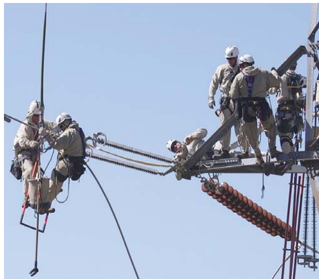
WAPA linemen replace dead-end insulators on a 230 kV tower using the energized HEC work method.
