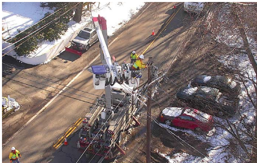
After major storms, FirstEnergy's in-house team of licensed pilots use drones to help assess damage—looking for downed wires, broken structures or problems challenging to detect from the ground.
