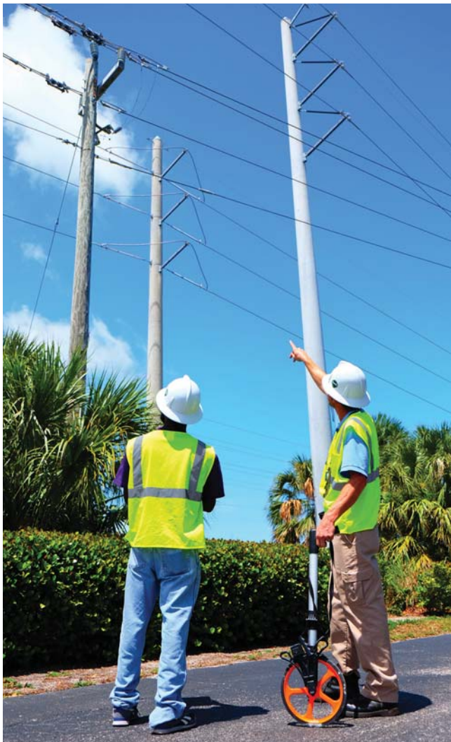
D & D Power, a division of BHI Energy, has hired retirees from National Grid and other local utilities to help in the training process with the younger linemen and apprentices.
