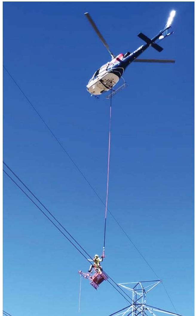
An LADWP crew member removes a spacing cart from the line after replacing double bundle spacers.
