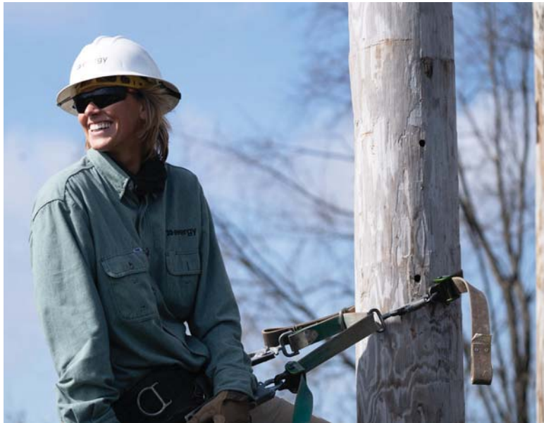
At MCC, Blaser taught her how to climb low and slow on the pole using a climbing belt and BuckSqueeze from Buckingham Manufacturing.
