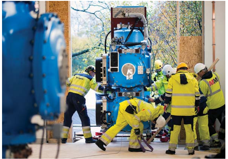
Team moves blue GIS from platform erected outside substation into building.
