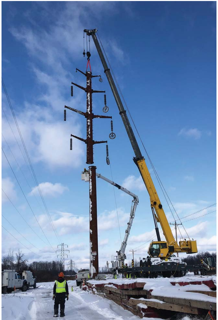
Three Phase Line crews use a mobile telescoping crane to assist in connecting a new Cor-Ten steel transmission tower near Cicero, New York, for National Grid.
