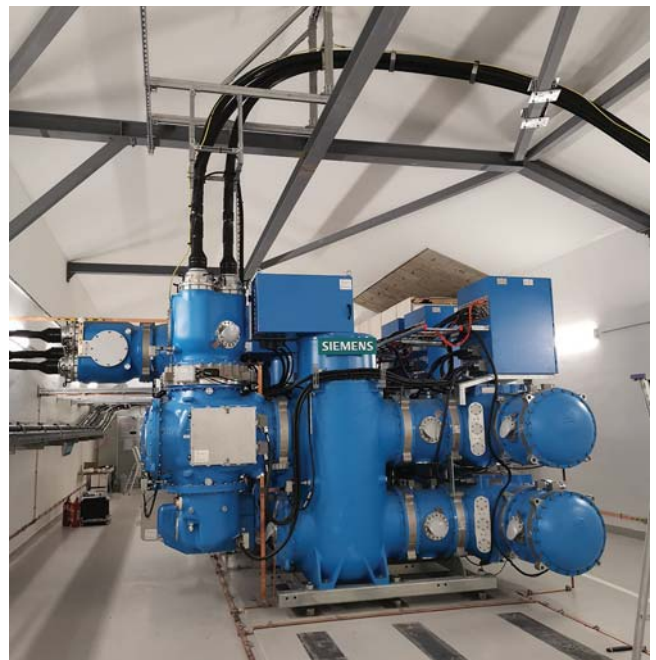
Blue GIS installed in switch room. Incoming cable is over blue GIS and transformer cables exit switch room through wall on left.
