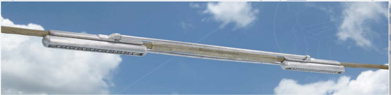
Transmission Splice Repair and Uprate
