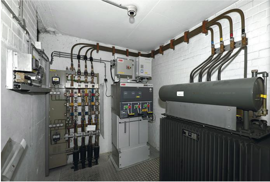
This is a typical Enexis medium-voltage/low-voltage indoor substation that includes a MV/LV distribution transformer, MV switchgear and a LV distribution board that has been upgraded to include distribution automation.
