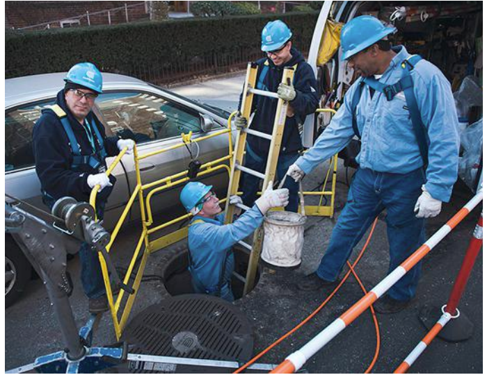
More than 833 miles of new cable was installed in the Con Edison service territory in 2015.
