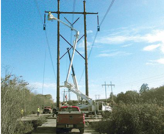
Crews string 345-kV conductor using swamp mats as work pads along the right-of-way.
