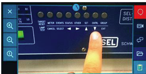
The Atheer Air O&M app consists of instructions, pictures and videos associated with settings change on an SEL 351A substation relay to put it into maintenance mode and then return it back to normal mode.
