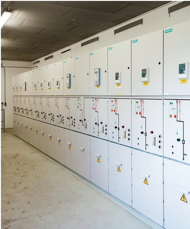
A medium-voltage switchgear installation equipped with distribution automation and protection relays, showing different relay and switchgear indications.
