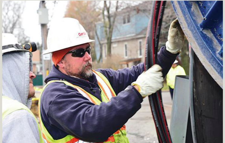
ComEd linemen work to replace underground distribution cable through a program enabled by the Energy Infrastructure Modernization Act.
