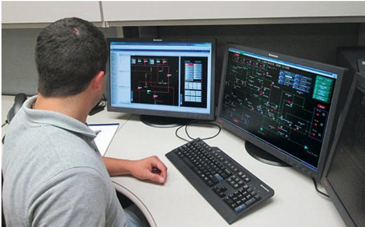
Westar Energy distribution automation engineers use HMI and SCADA screens to maintain the DA system as well as interfacing and commissioning new equipment being deployed to the field.
