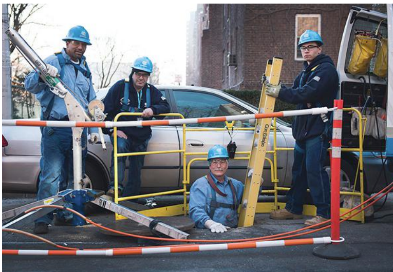
A Con Edison crew replaces underground secondary-cable in Lower Manhattan.
