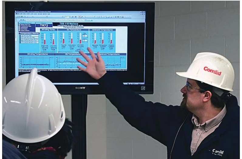
Data collected from sensors in intelligent substations will allow engineers to use predictive algorithms to better direct maintenance activity.
